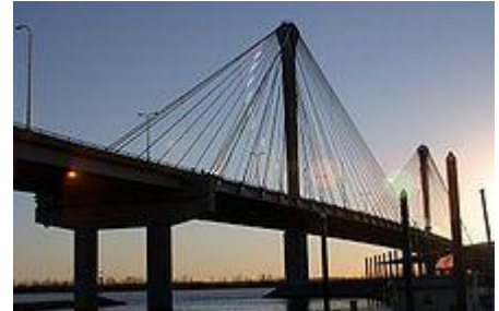
The Clark Bridge is a cable-stayed bridge across the Mississippi River between West Alton, Missouri and Alton, Illinois.
